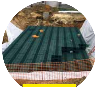
Rigofill inspect 📍 Clairefontaine (78)
